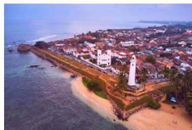
Galle is known for stunning beaches, the ancient Galle Fort and Galle Lighthouse
